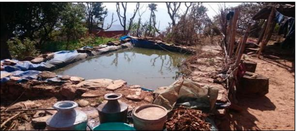
Fig: - 39 A plastic pond was made at Okhaldhunga to harvest the rain water.
